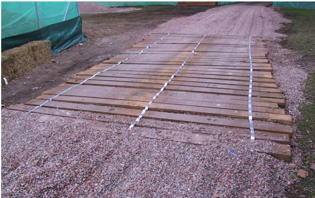
Figure 19 – Example of acceptable Tree Protection Area ground protection
