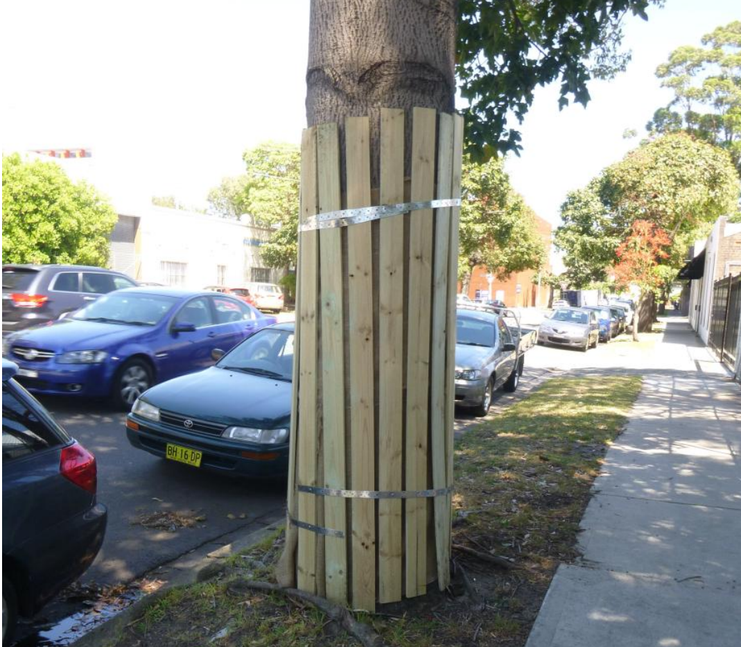
Figure 20 – Example of acceptable Trunk Protection batten installation
